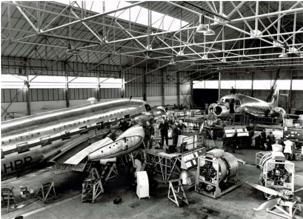
A view inside the maintenance hangar at Northolt with Viking 1B G-AHPP and another undergoing comprehensive works. Bristol Hercules powerplants are waiting in their stands in the right foreground. While the earliest Vikings started life with an outer wing design based on that of the Vickers Wellington with geodetic construction, they were soon replaced with more conventional all metal mainplanes. (BEA photo 3249)
