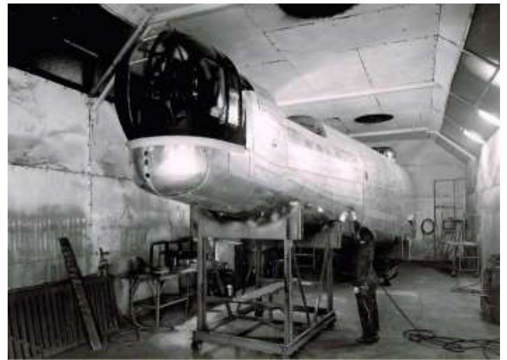
Above Left; The Chrysler Motors Limited, Kew Works. Above Right; The Chrysler Motors paint shop, with a complete rear half of a Halifax fuselage in place for painting.
