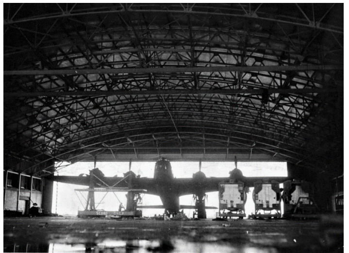
Above Left; The twin tail wheels which were a feature of every Stirling and are obvious in this photo. Above Right; How closely the 99-foot wingspan of a Stirling fitted into a standard pre-war built RAF hangar can be seen in this 1942 photo.
