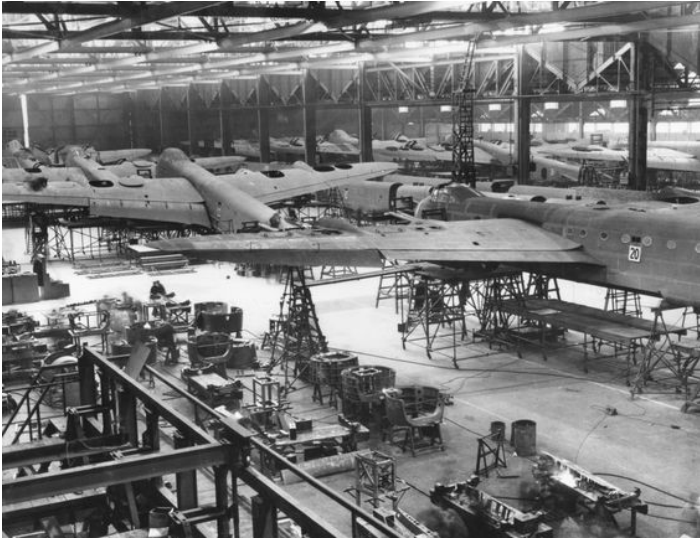
Above Left; Mass production of Stirlings underway. Above Right; A further photo of Stirling production. Note the cabin windows that were thoughtfully provided for when aircraft were used in their secondary passenger/ trooping role.
