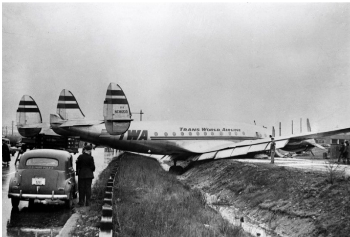
Above Left; NC86510 “Star of Rome” was damaged beyond repair in this accident at Washington National on 29 March 1946. Following a landing on a wet runway it continued over the end of the runway, struck an airfield building and ended in the ditch as seen above.
